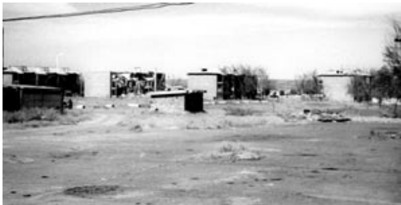
Figure 1. View of Mirnyi, formerly a mining town, but now a ghost town located about 40 km west of Lake Balkhash. Despite clear signs of decline, which is also evident in the surrounding Kazakhstania province, it still provides shelter and infrastructure for fieldwork.
