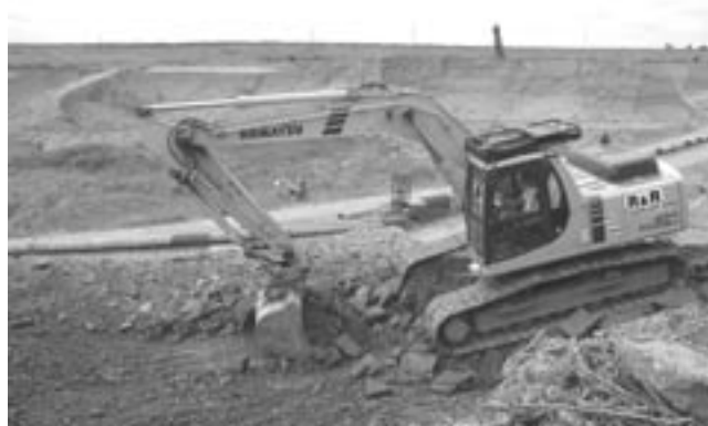
Overburden removal in action!
