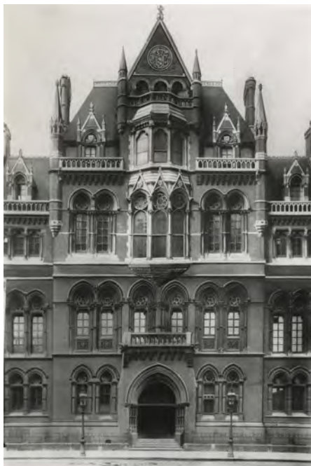
Neo-gothic frontage of the Mason Science College. The original departmental geology museum occupied the very top floor, lit by two large skylights flanking the steep central peak. Image courtesy of Cadbury Research Library.
